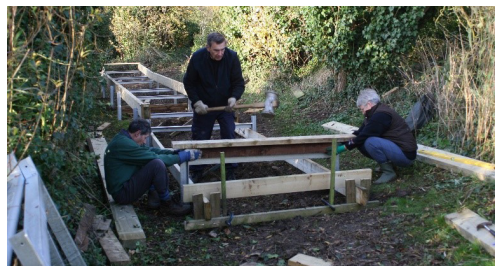
The construction of the Boardwalk in 2009 Photos: Nigel Sprowell
